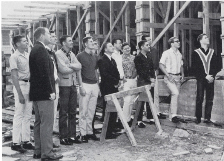
Club members observe construction on the school's new wing.
